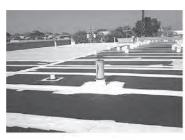
colors. When installed in white, #6000 will reduce theroof's surface temperature which reduces stress from daily heat cycles. It will also reduce the heat gain in the building's interior, any associated air conditioning costs and increase the efficiency of roof mounted air conditioning condensers.
