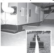
The Quick Block is designed to replace the current practice by skilled trades people of building wooden blocks for support of vital mechanical infrastructure on flat roofs including:
