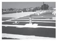
colors. When installed in white, #6000 will reduce theroof's surface temperature which reduces stress from daily heat cycles. It will also reduce the heat gain in the building's interior, any associated air conditioning costs and increase the efficiency of roof mounted air conditioning condensers.
