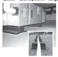
The Quick Block is designed to replace the current practice by skilled trades people of building wooden blocks for support of vital mechanical infrastructure on flat roofs including:
